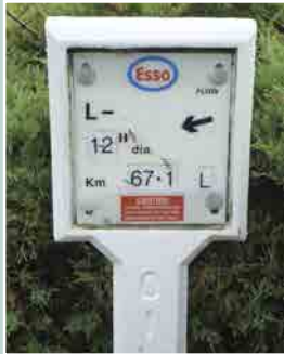
Esso marker posts
