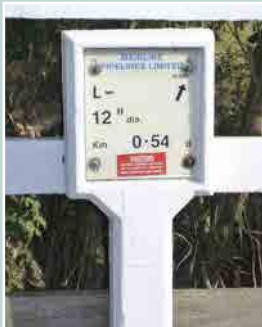
Mainline marker post
